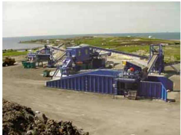
The SYSAV sorting site for bottom ashes at the Spillepeng landfill in Malmö. Photo: SYSAV
