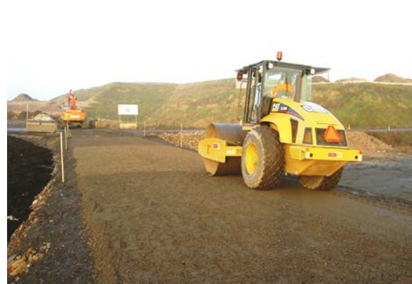
Figure 4. The test road in Malmö comparing virgin base gravel (light brown area) with SLAGASPHALTbase.
