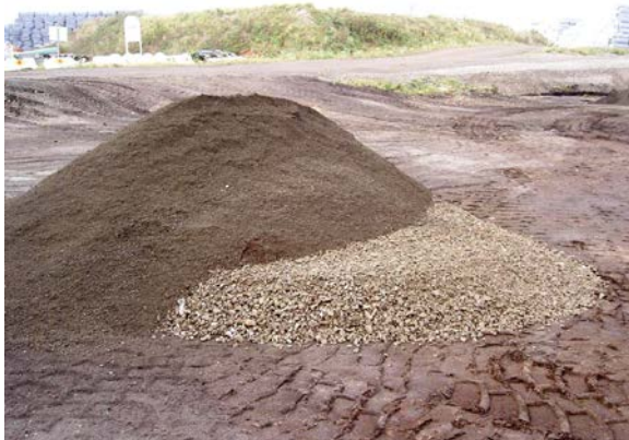
Figure 3. A prepared blend of SLAGsand and ASPHALTgravel on top of ROCKgravel before mixing it all together.
